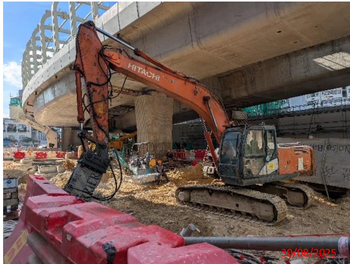
Remark 2: Site photo of noise mitigation measure
