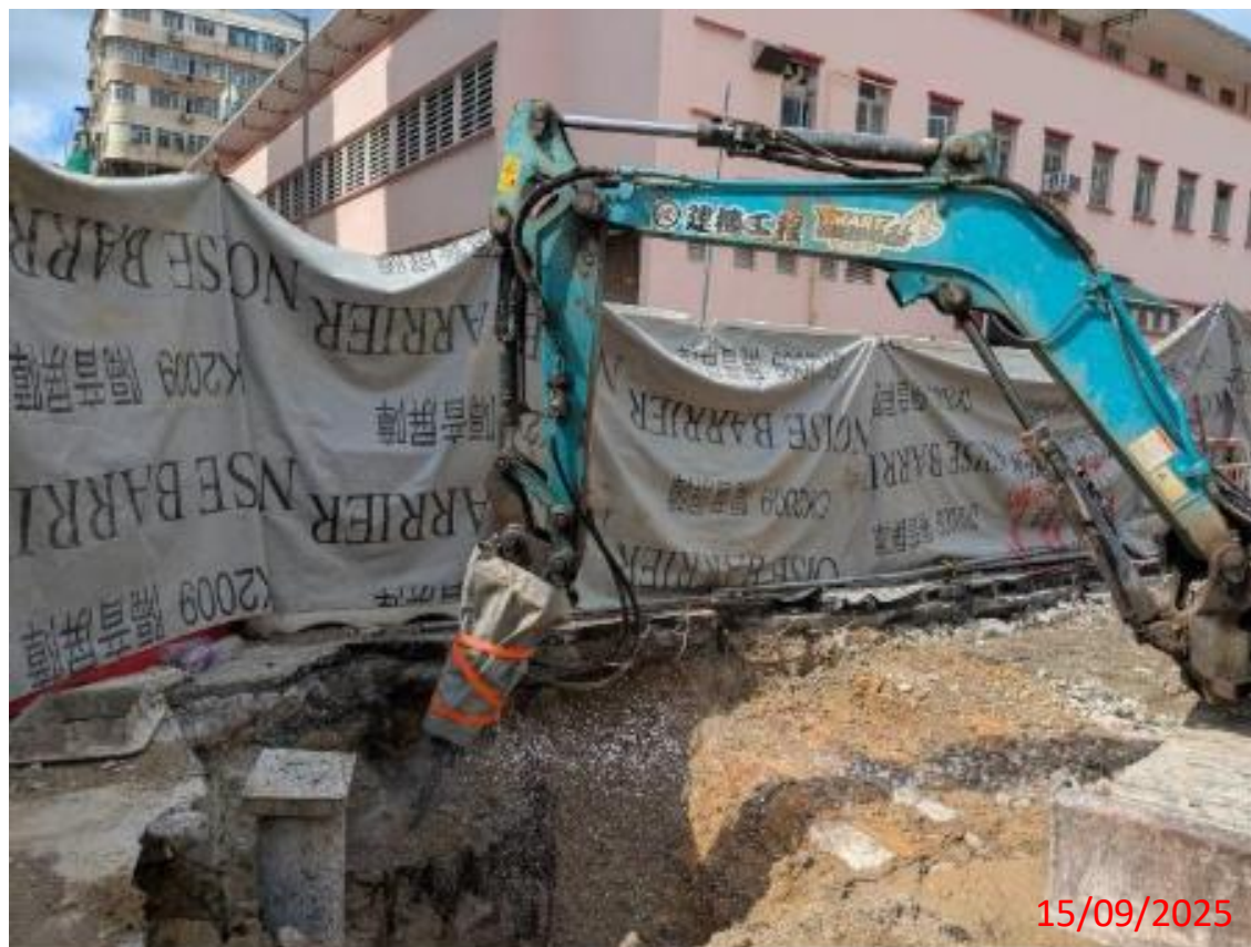
Remark 2: Site photo of noise mitigation measure
